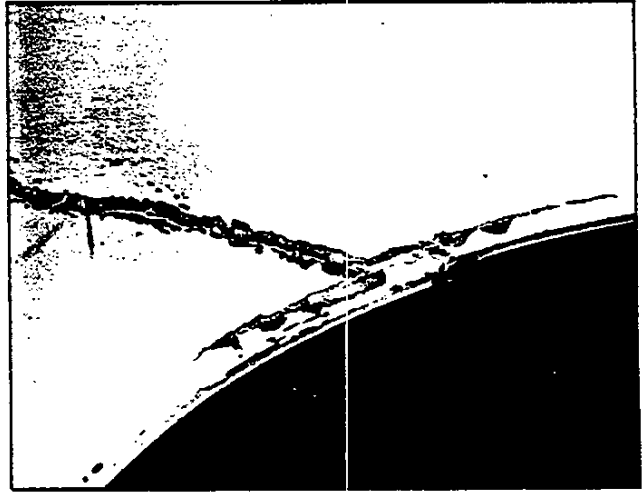
Fig. 58—Typical Cracked Panel
